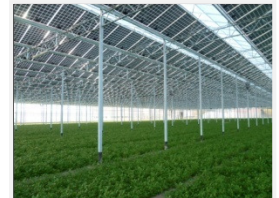
Greenhouse solar PV
